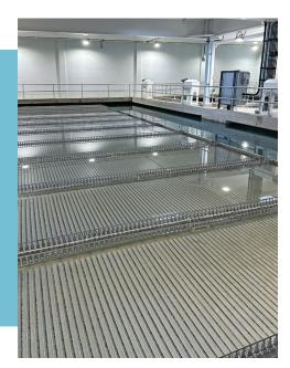
↑ The new Inclined Plate Settlers separate out the clumps of "floc" particles formed in the flocculation basins. This water is now ready for disinfection and filtration.
