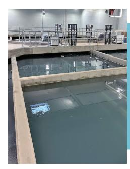
↑ In the Flocculation Basins, sediment and suspended particles in raw lake water are chemically bound together to facilitate their removal.
