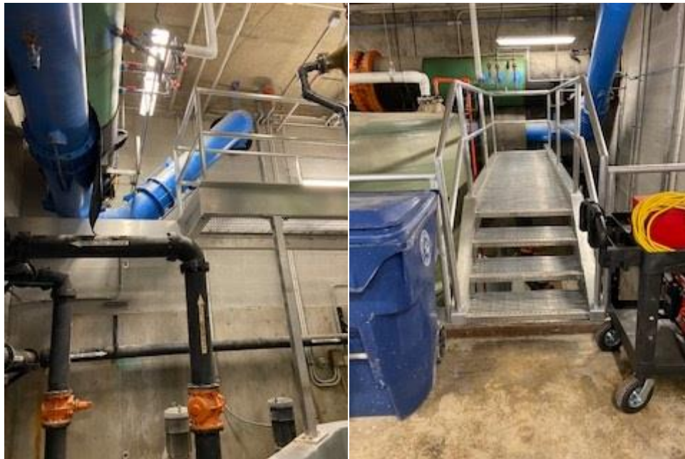
North Settled Water Maintenance Access Platform
