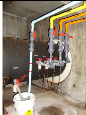
Filter Backwash Recycle Line
