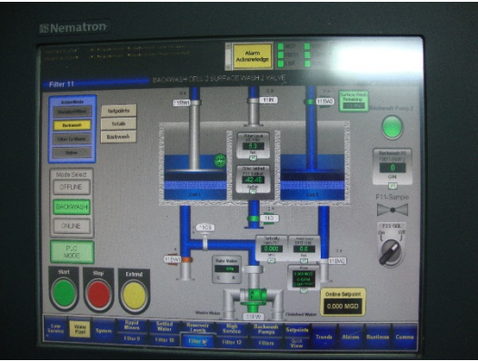
Filter #11 and #12 Control Console HMI
