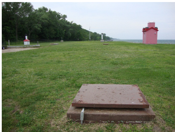
0.9 MG Reservoir (foreground) 1.8 MG Reservoir(background)
