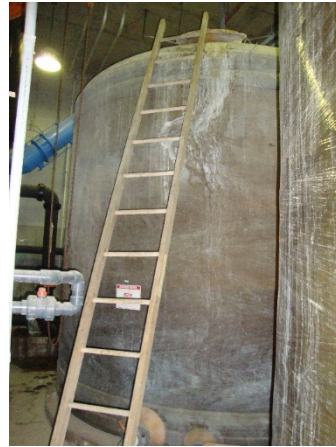
Secondary Alum Feed Point Into 30-Inch Raw Water Main
