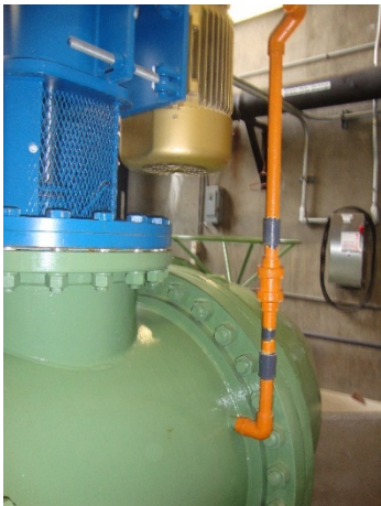
Primary Alum Feed Point Into Rapid Mixer
