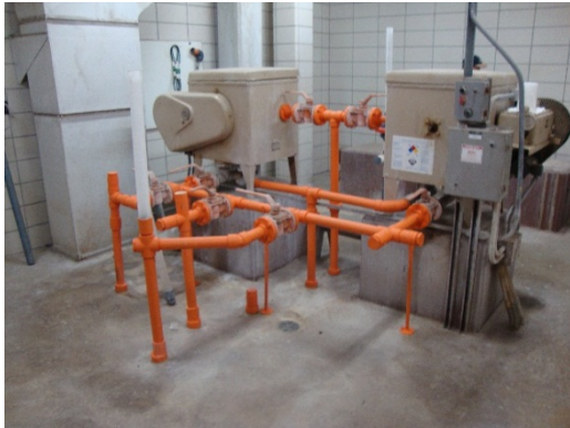
Rotodip Feeders
