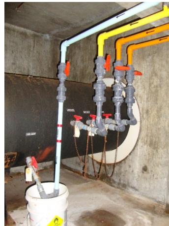
Secondary Alum Feed Point Into 30-Inch Raw Water Main
