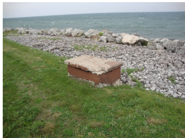
Vent Structure on 0.9 MG Reservoir
