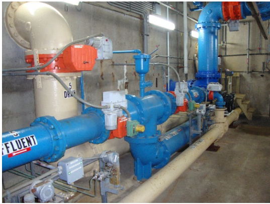
Filter #5 Effluent Piping
