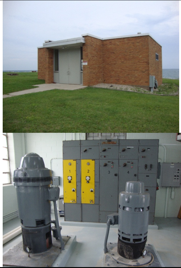
South Low Lift Pump Station
