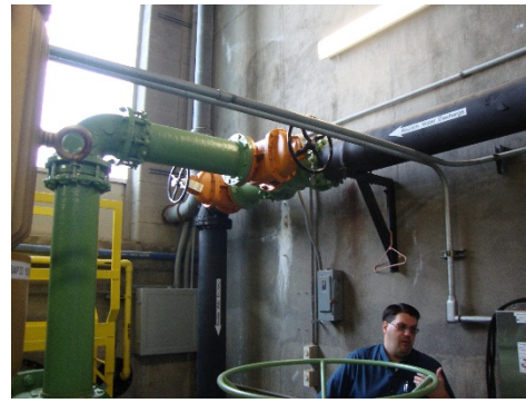
Filter Backwash Recycle Line
