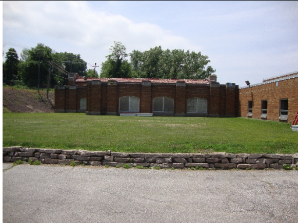
Old Underground Sedimentation Basin
