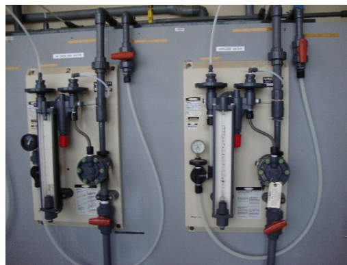
V-notch chlorinators
