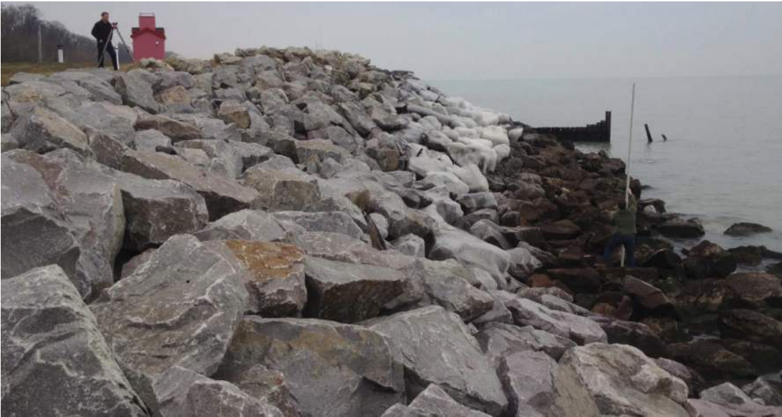
Figure 38: St. Joseph Water Plant Revetment, spring 2012
