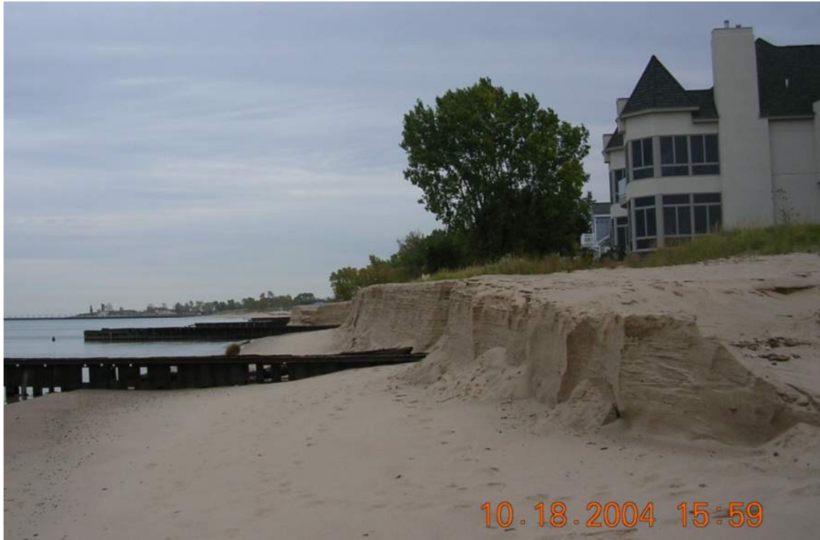
Figure 21: October, 2004 - Area 2 short term erosion
