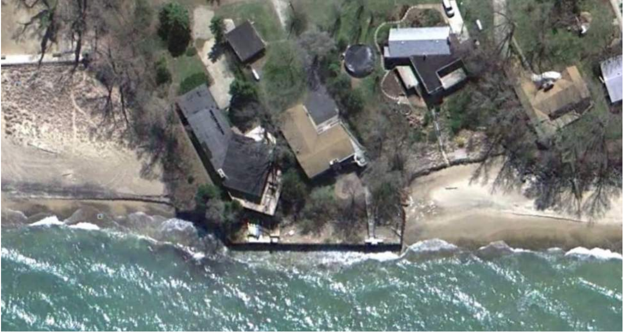
Figure 34: Example of flanking in southern Berrien County. Note how this failure has resulted in the loss of the public trust property lakeward of the structure and public passage is only possible in the lake itself.
