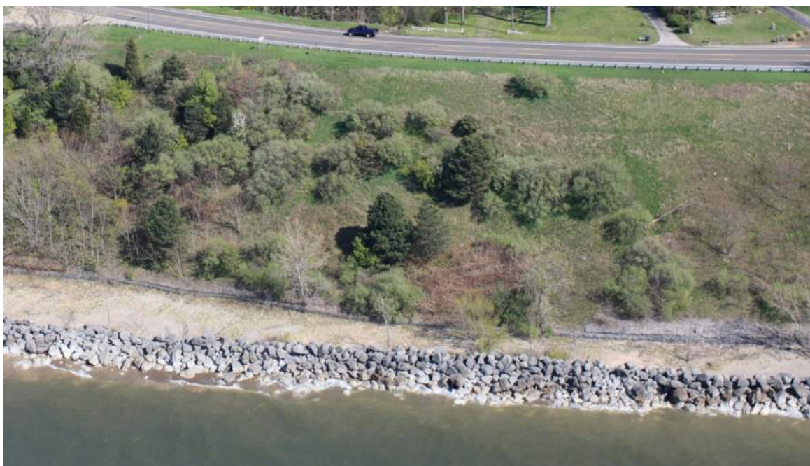
Figure 39: Stone Revetment along South Lakeshore Drive Oblique Photo
