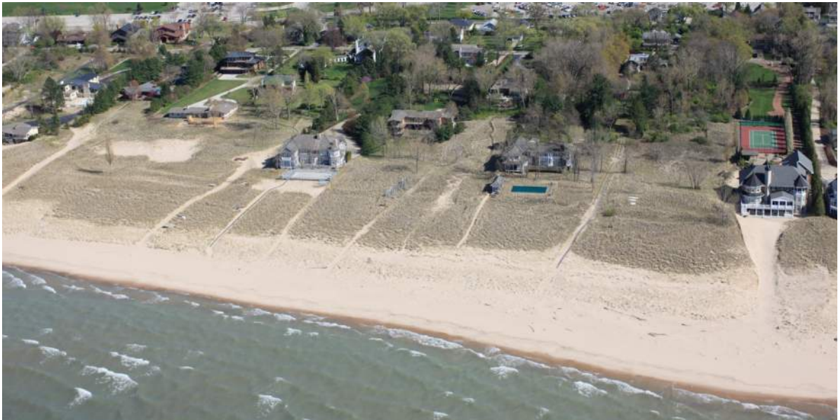
Figure 43: Area 1 typical shoreline during a low water condition (2012 USACE Oblique photo)
