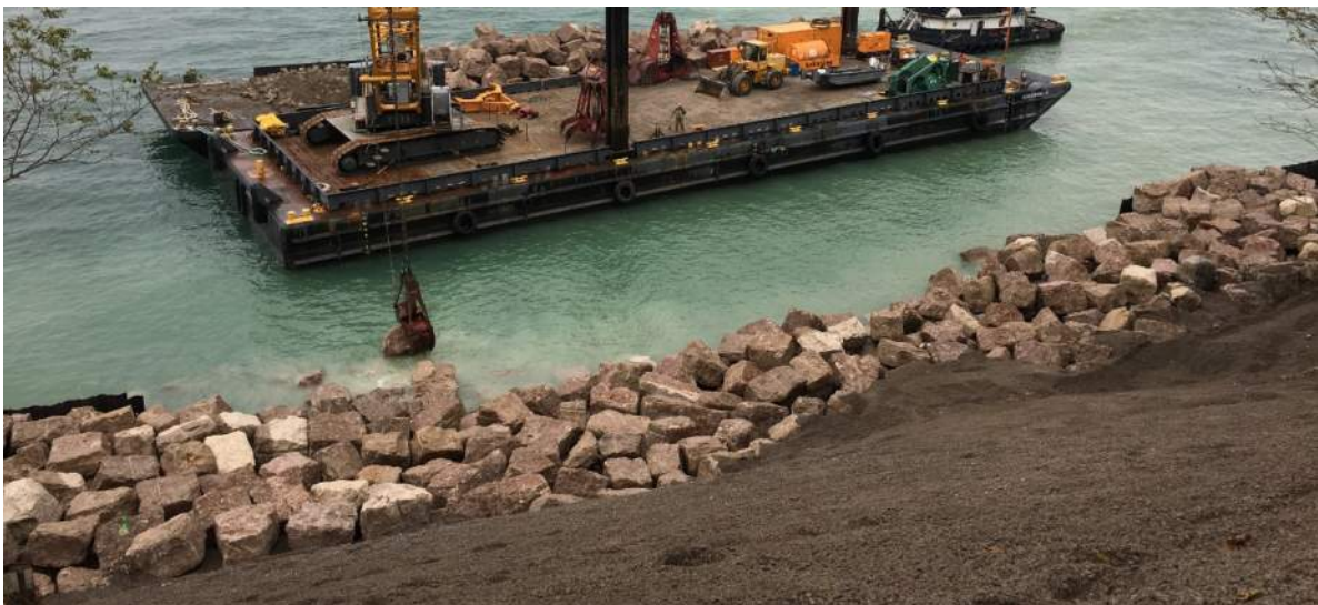
Figure 54: Area 3 CSX Shore Protection Project – placement of armor stone
