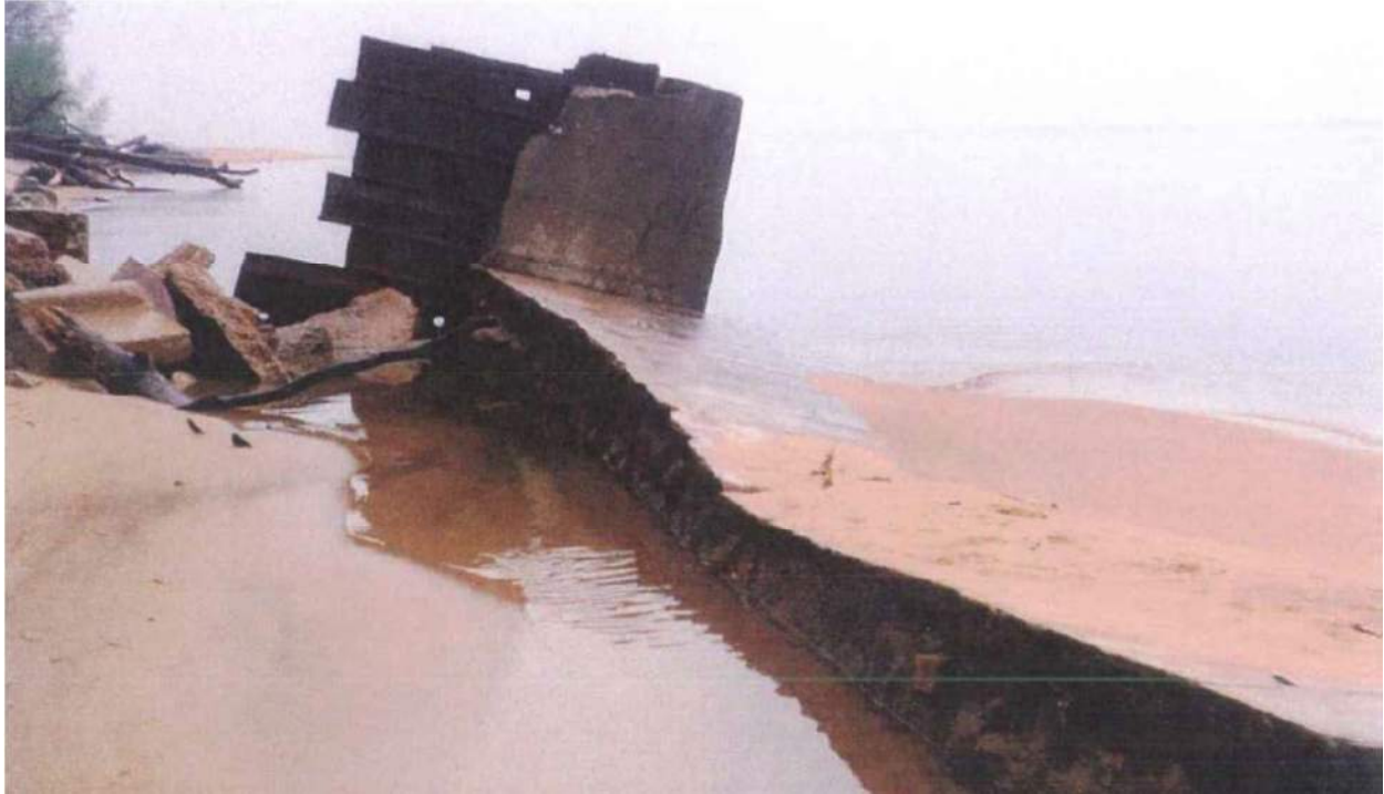
Figure 35: USACE CEM Photo, “A toppled concrete seawall along the Lake Michigan coast of Berrien County. Failure probably resulted from undermining of the underlying glacial till foundation, April 1991.”
