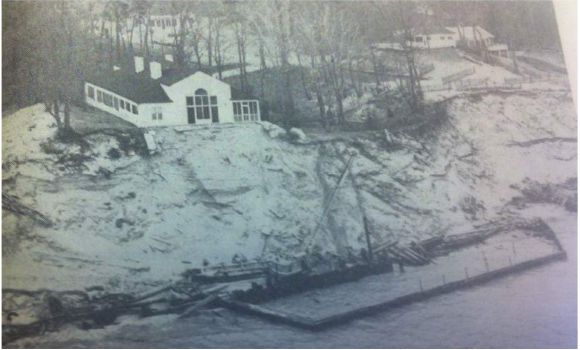
Figure 28: 1970s Herald Palladium photo of bluff erosion south of St. Joseph, MI
