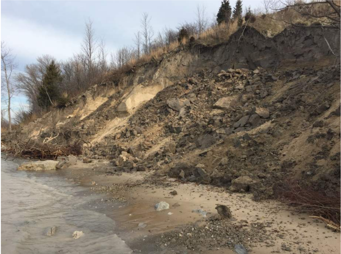
Figure 55: Area 3 – cohesive bluff erosion
