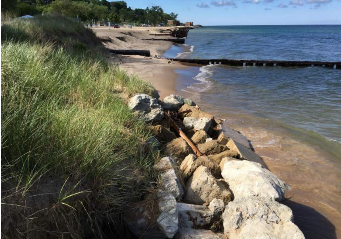
Figure 50: Area 2 Existing Shoreline Protection (Looking South)
