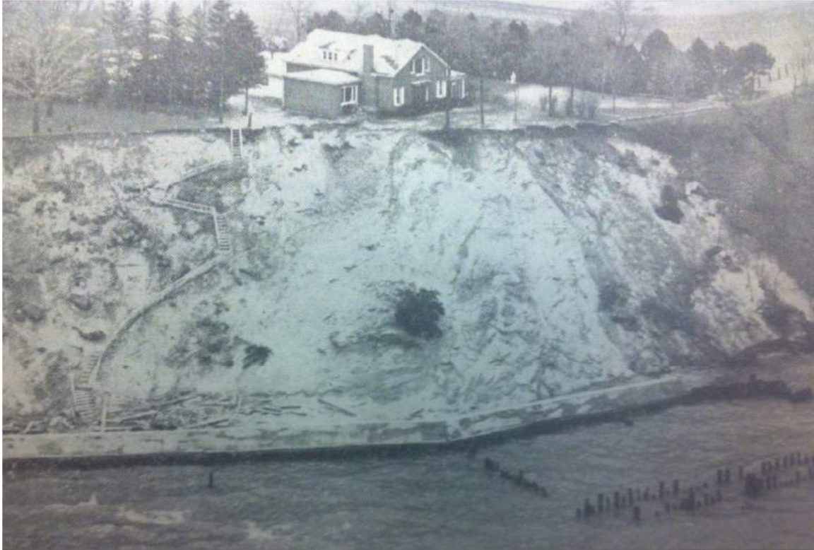
Figure 29: 1970s Herald Palladium photo of bluff erosion south of St. Joseph, MI
