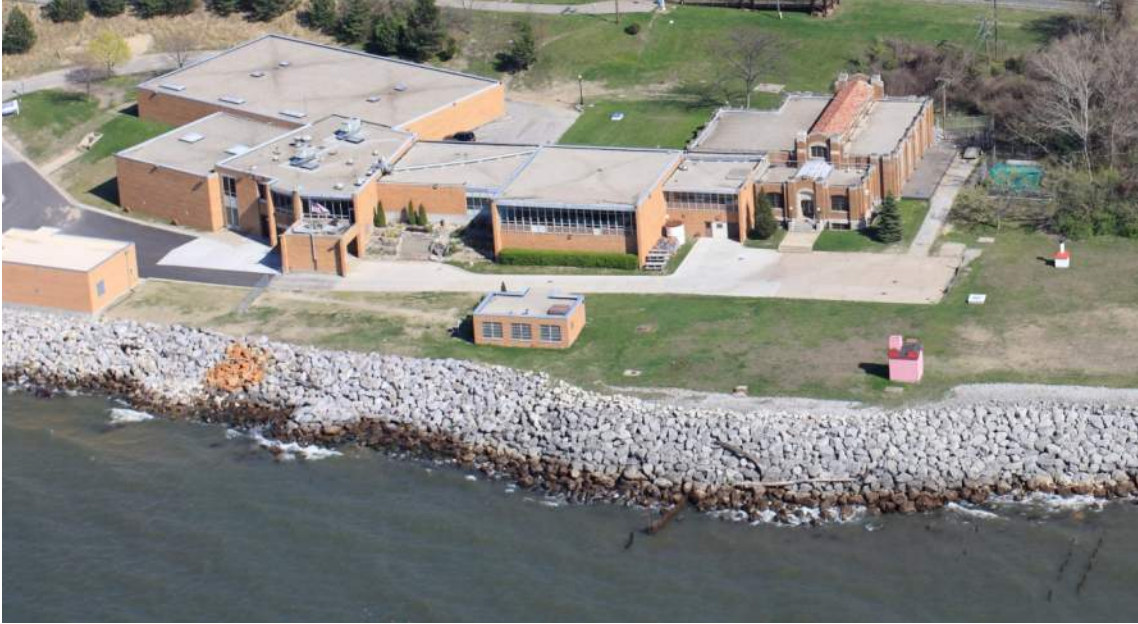
Figure 37: St. Joseph Water Plant Revetment Oblique Photo (U.S. Army Corps of Engineers)
