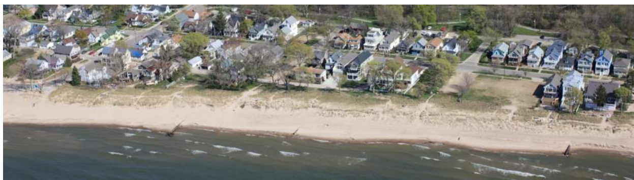
Figure 48: Area 2 typical shoreline (2012 USACE Oblique Image)
