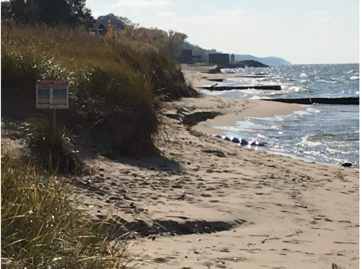
Figure 20: November, 2017 - Area 2 foredune erosion
