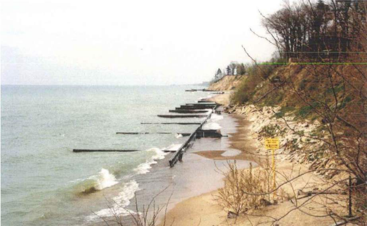
Figure 36: USACE CEM Photo, “A steel sheet-pile wall and groin field has been ineffective at protecting this section of cohesive shore along the Berrien County shore of Lake Michigan, south of the town of St. Joseph, April 1994.”
