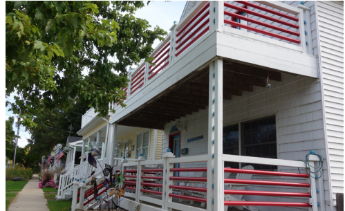
Homes within the Lions Park Neighborhood are generally older than homes in other areas of the City, with a significant number recently remodeled. These fall within the Single Family Residential Land Use category.
