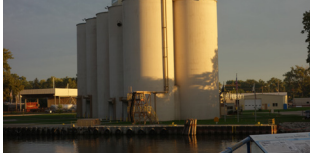
Lafarge is an existing industrial land use.
