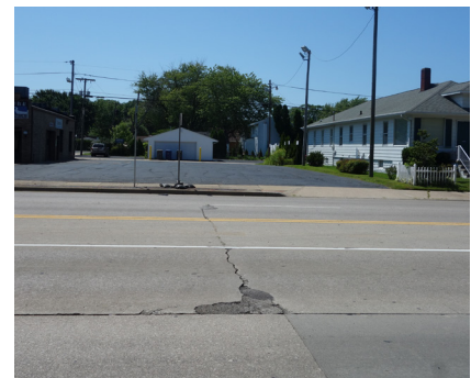
Because of limited funding, pavement condition in St. Joseph has deteriorated in recent years.
