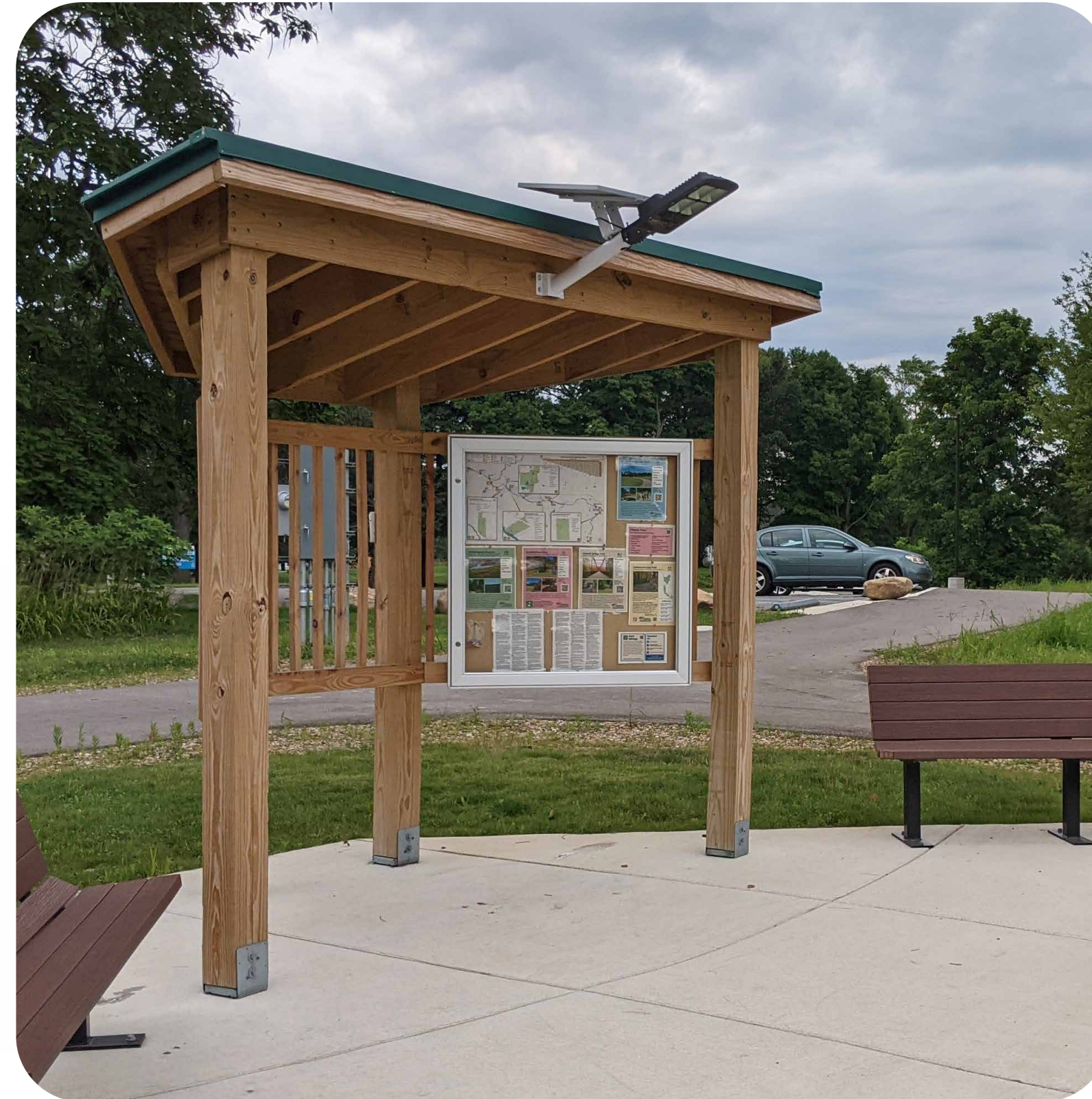
Information kiosk, security lighting, and bench at trail head and/or kayak launch
