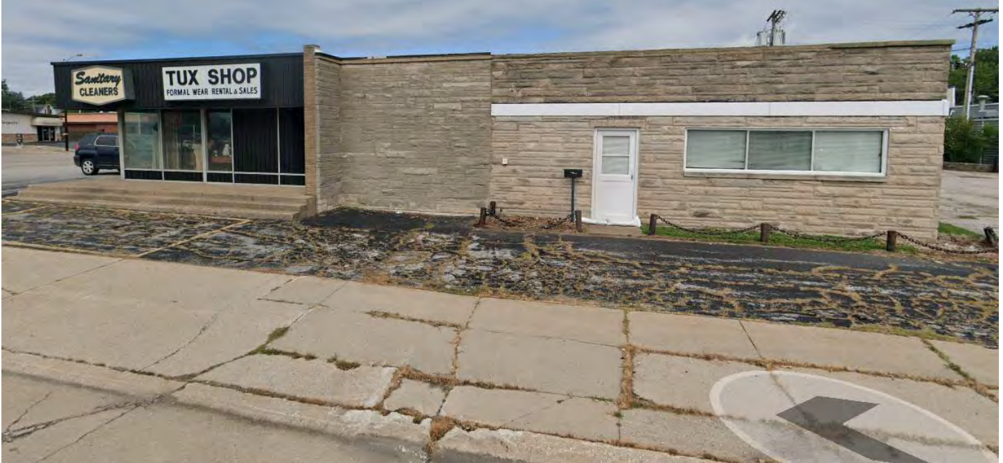
Photo credit: Google Street View
