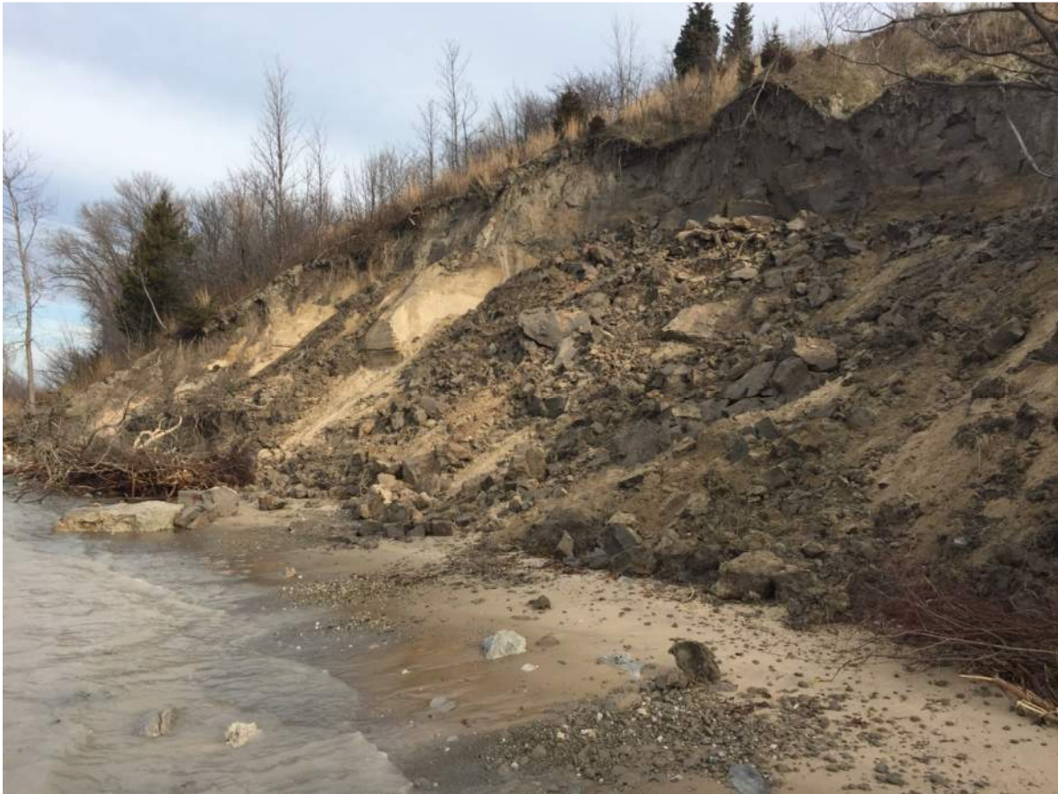
Figure 55: Area 3 – cohesive bluff erosion
