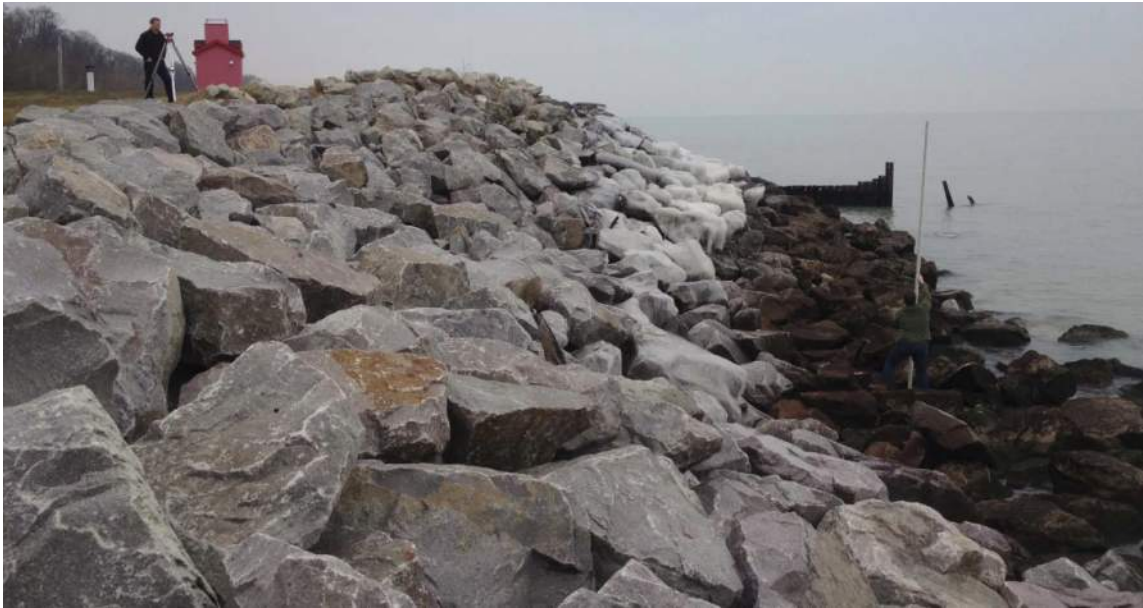
Figure 38: St. Joseph Water Plant Revetment, spring 2012
