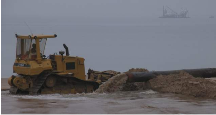
Figure 18: 2012 photo of beach nourishment south of Park Street showing the dredge in background
