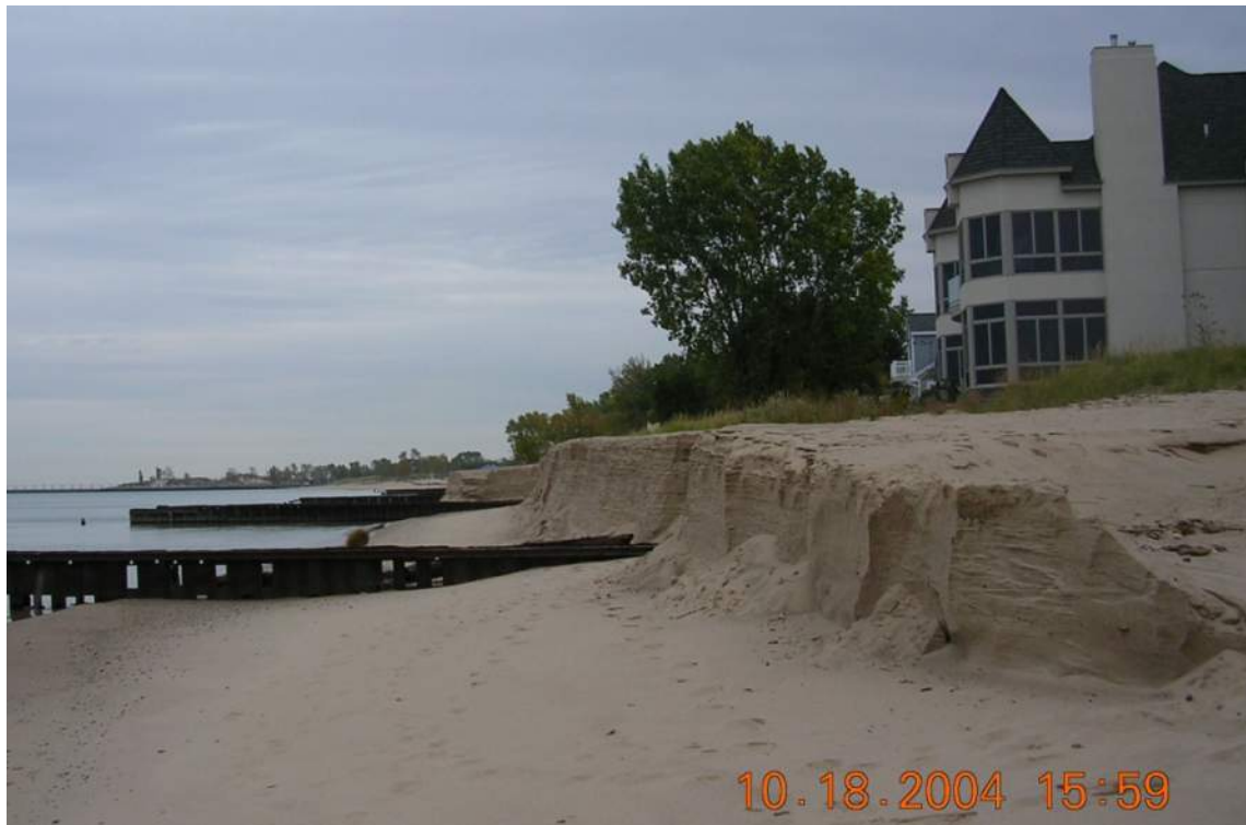
Figure 21: October, 2004 - Area 2 short term erosion
