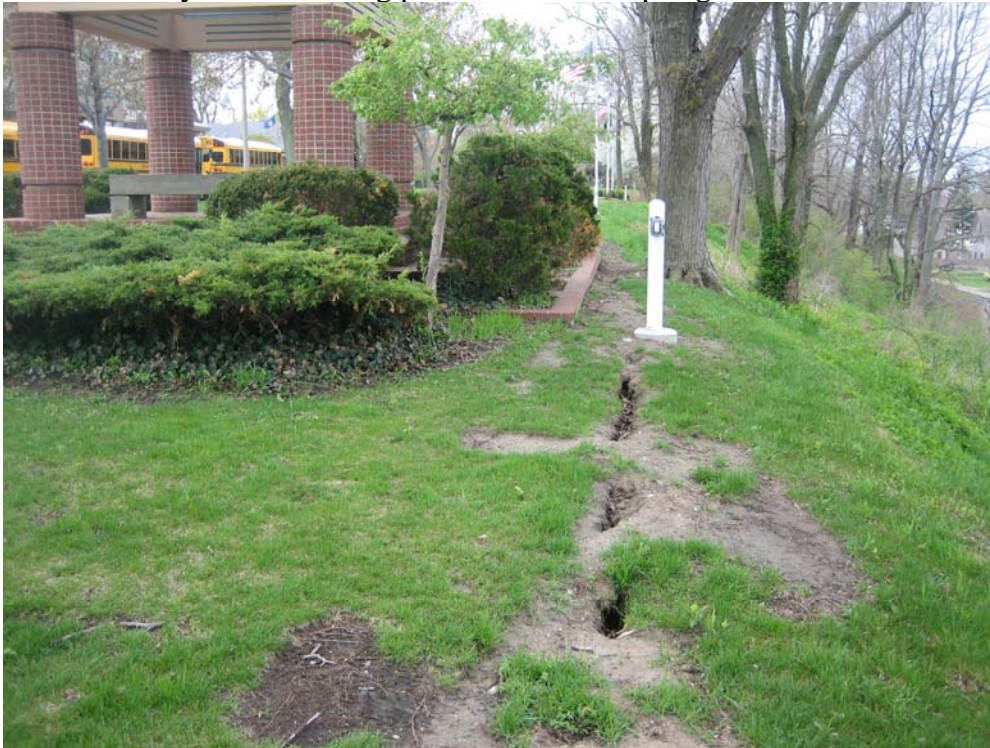
PHOTO NO. 13: Looking northeast along the top edge of the bluff. Note the scar from the utility trench running parallel with the top edge of the bluff.
