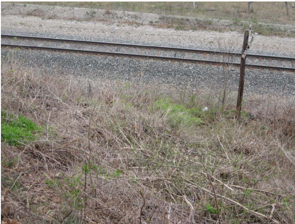
PHOTO NO. 42: Looking northwest down the bluff face. Note the brush that has been cut.
