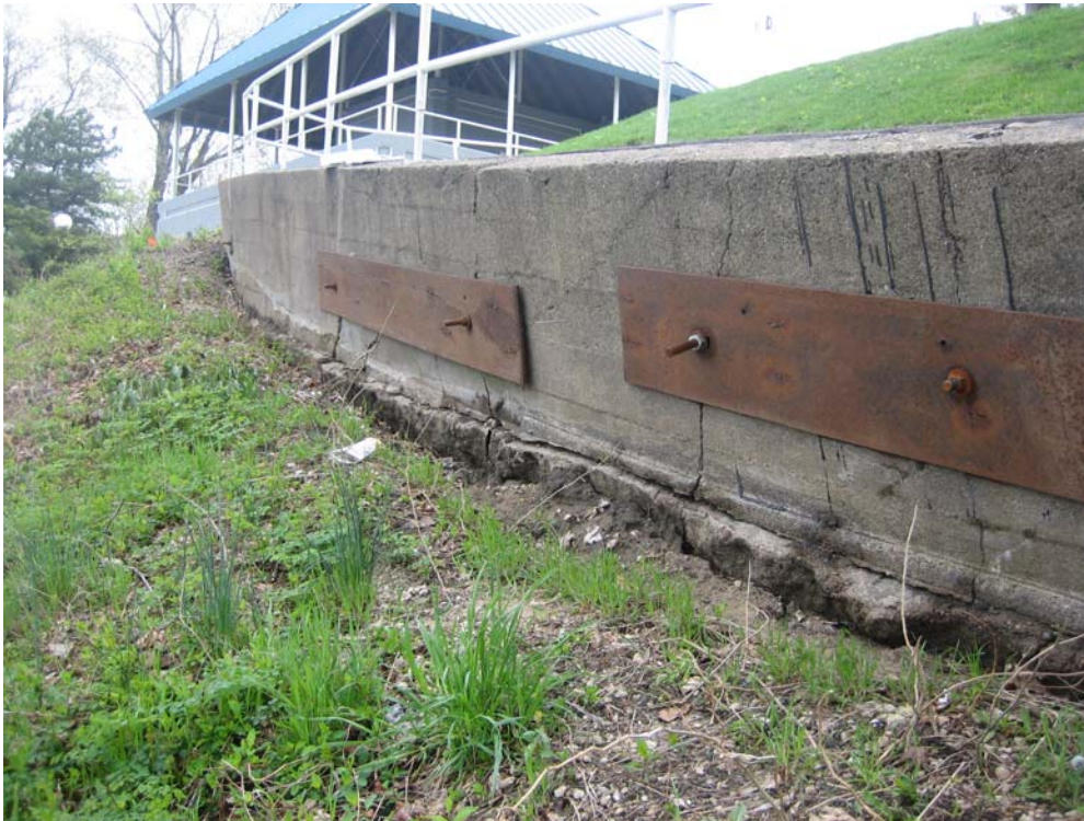
PHOTO NO. 17: Looking northeast at the upper portion of the walkway retaining wall. Note the steel plates and anchorages.
