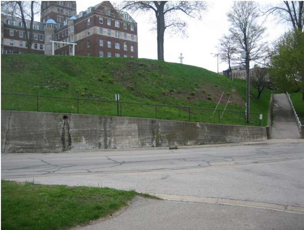
PHOTO NO. 31: Concrete retaining wall along Water Street near base of walkway. Note water stains at drain discharge location.
