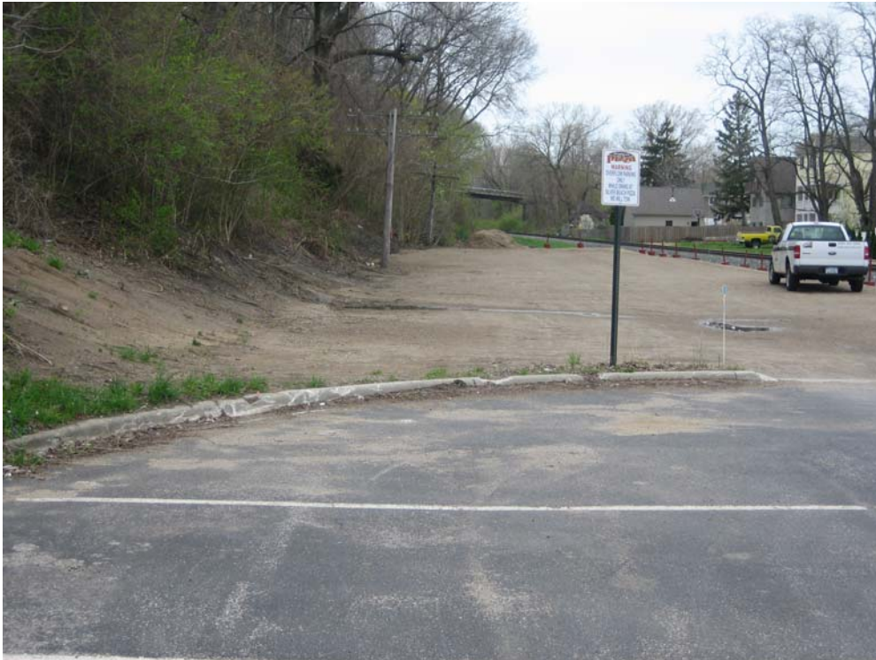
PHOTO NO. 9: Looking southerly along the base of the bluff.
