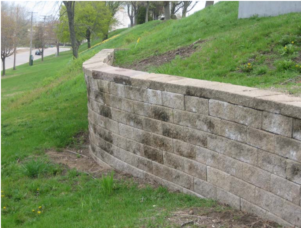
PHOTO NO. 25: Upper MSE wall looking northeast.
