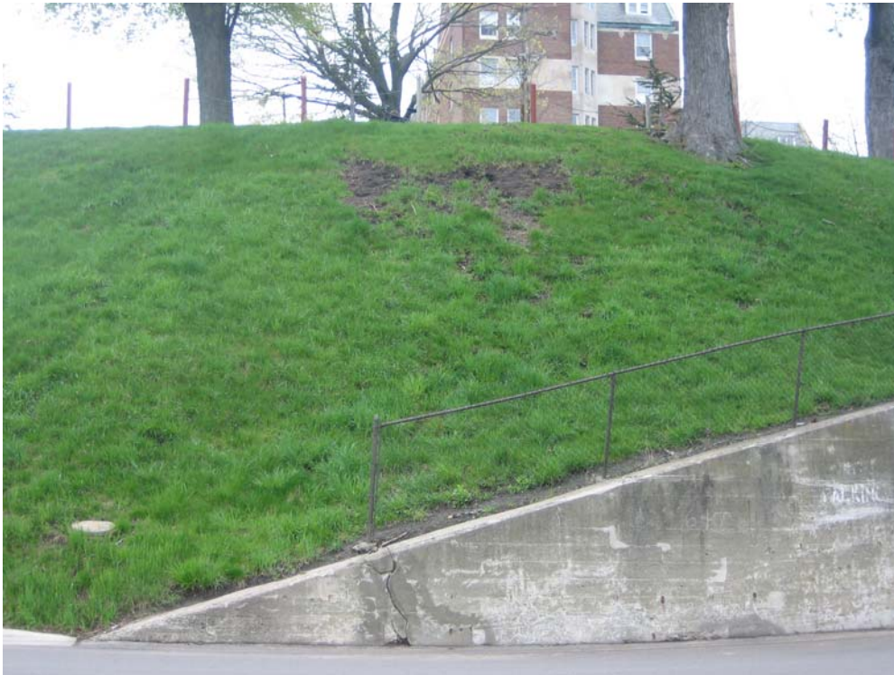
PHOTO NO. 35: Note cracking near the end of the concrete wall and erosion along grassy slope face.
