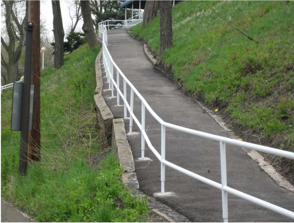
PHOTO NO. 19: Looking northeast up the walkway. Note the retaining wall movements.
